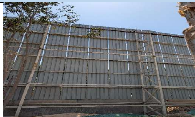
WIND BREAKING WALLS
